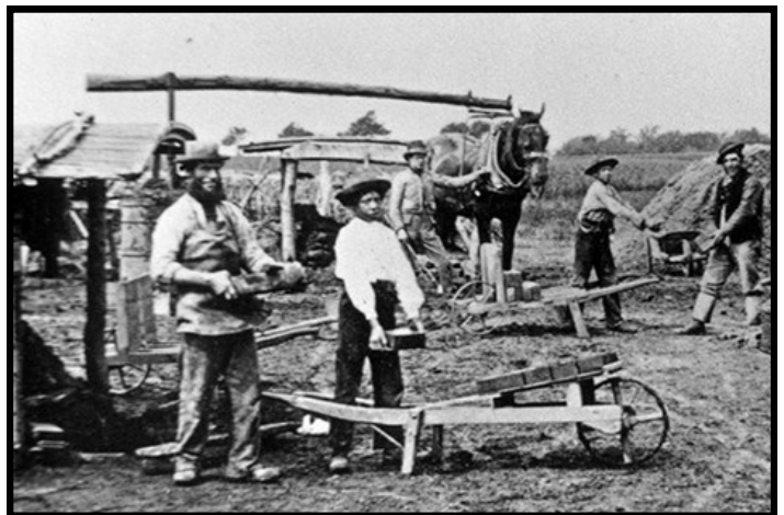
Horse-powered ring-pit for mixing clay for bricks or pottery manufacturing. England.
