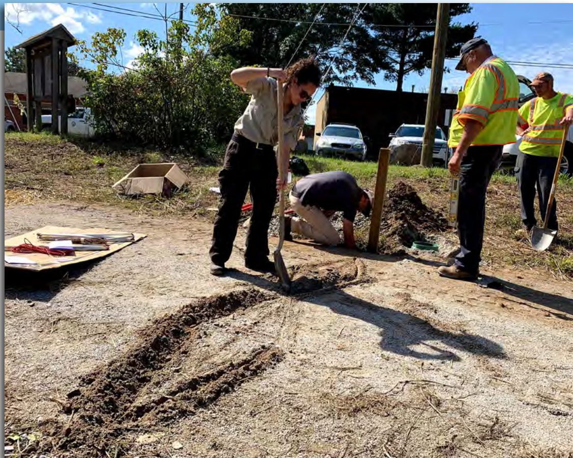
USFWS Visitor Services Specialist Carina Velazquez-Mondragon digs a shallow trench for the new eco-counter at Occoquan Bay NWR.
