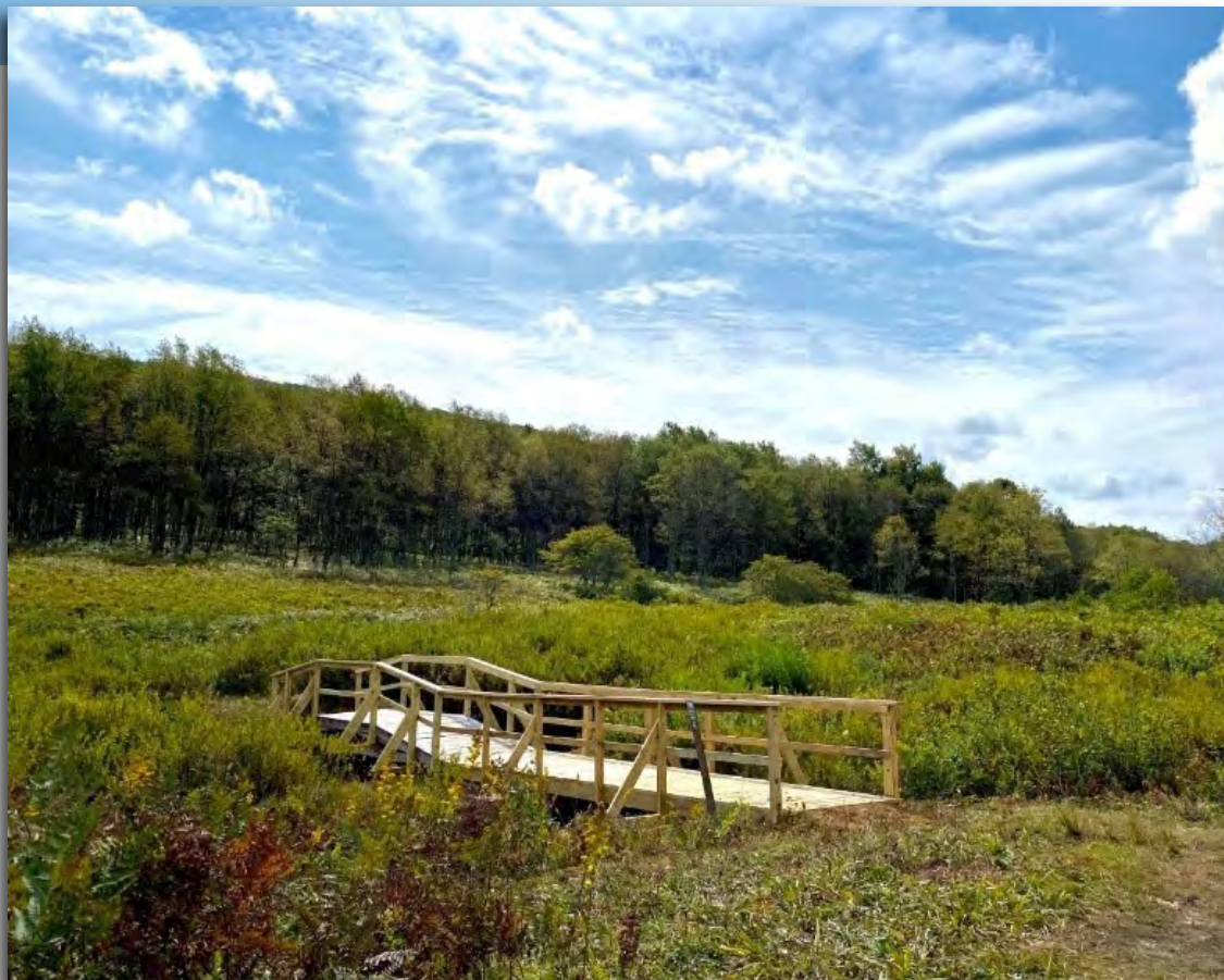
Elevated boardwalk built across Glade Run Stream.
