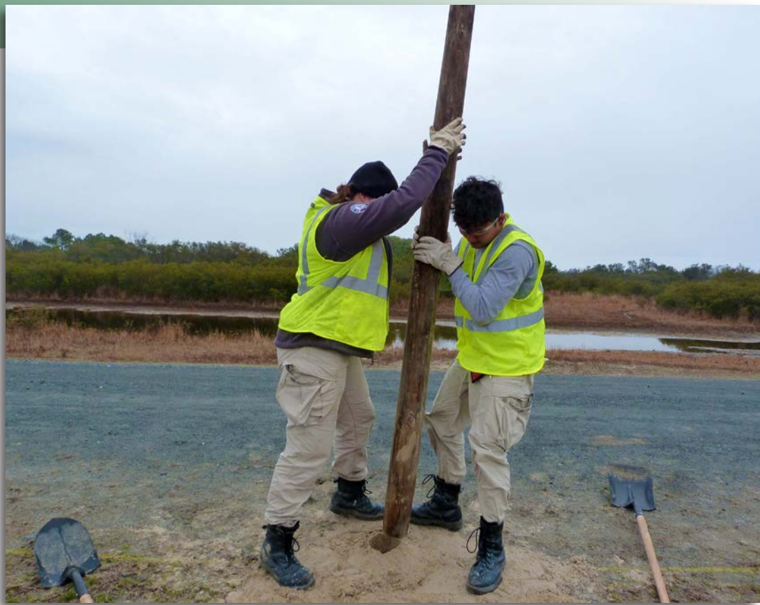
AmeriCorps members install a fence post USFWS
